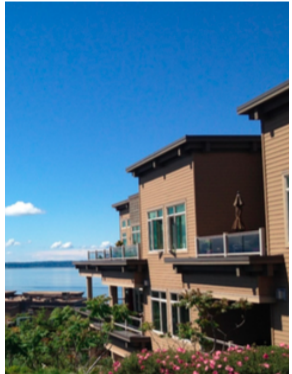
Point Edwards Community Photo credit: Sweek Consulting Engineers, LLC
